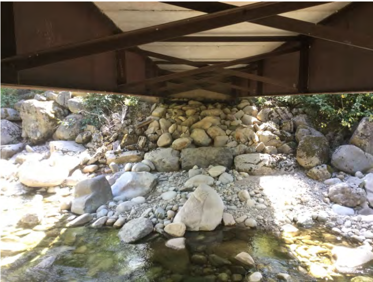
Left Bank Abutment when facing downstream
