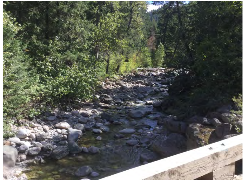
Upstream from Crossing
