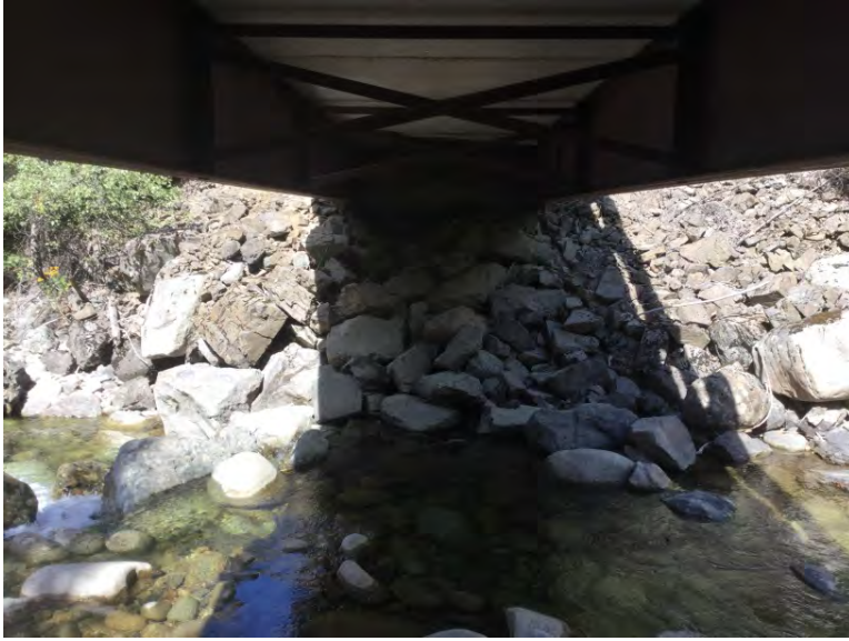
Right Bank Abutment when facing downstream
